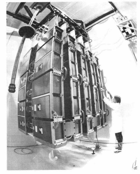
LARRY SCHNEIDER (1251) inspects a Marx Generator designed by the PBFA-II project team, of which he is a member. Thirty-six similar generators will form the energy storage section of the Labs' Particle Beam Fusion Accelerator-II, scheduled to begin operation in 1986. The nine-foothigh units will be capable of delivering a six-million-volt pulse of energy in a millionth of a second. Photographer Russell Smith (3155) took the photo with a fish-eye lens, which accounts for the distortion.
